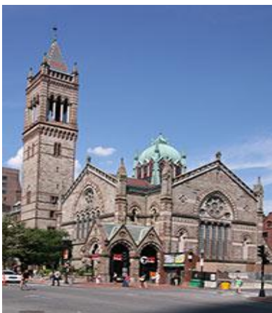
"NEW" OLD SOUTH CHURCH Willard T. Sears , Architect
