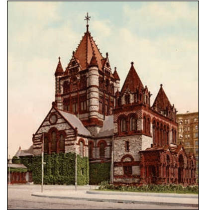
Trinity Church (completed in 1877) Copley Square, Boston, Mass.
